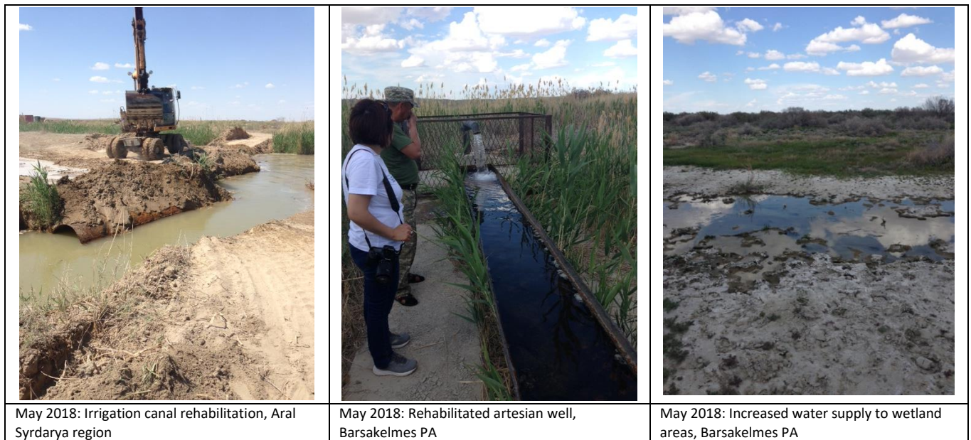
Figure 8: Photographs of rehabilitation of irrigation canal and rehabilitated artesian well
